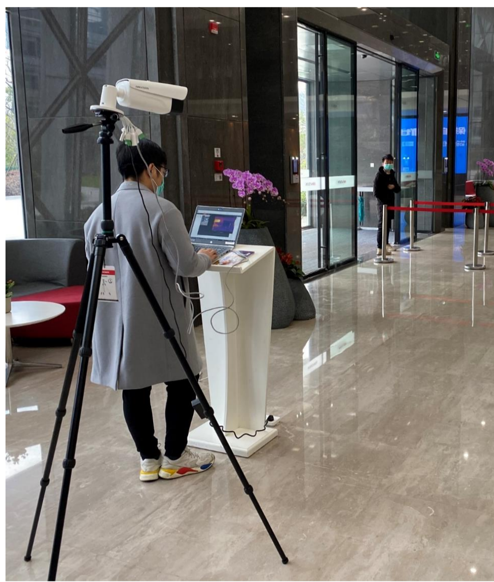
D. Installation complete
