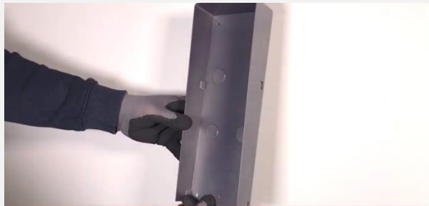
It improves the IP protection when the door station is placed on uneven brick walls and prevents rain drops from obstructing the camera lens
